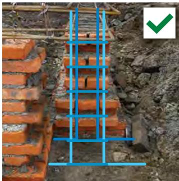
在构造柱处,砌砖基础应建有马雅槎。构造柱中钢筋应该延伸至砖基础底部,端部弯勾长度至少36cm。The long bars from the column should extend to the base of the foundation and terminate with anchors that are at least 36cm long.
