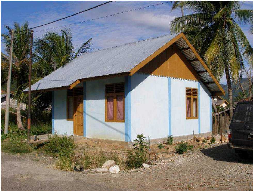
Figure 4.3. Confined masonry house constructed by Build Change and Mercy Corps in Banda Aceh, Indonesia
