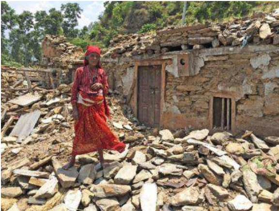
Figure 3.24. Devi Timilsina in front of her collapsed house
