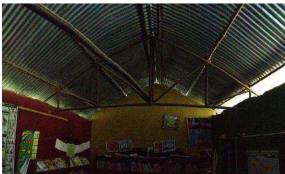
Figure 4.4. School in Dhungkharka with steel framing
