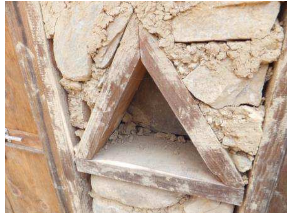
Figure 3.30. Wall opening for shrine, Dhungharkha
