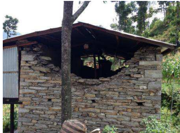
Figure 3.11. Stone wall construction, Ramche, Sindhupalchok
