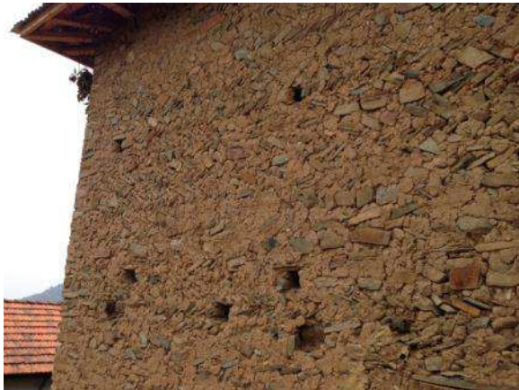
Figure 3.10. Stone wall construction, Chalal Ganeshthan, Kavrepalanchok
