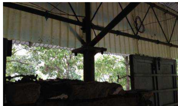
Figure 4.5. Steel framed school in Ramche
