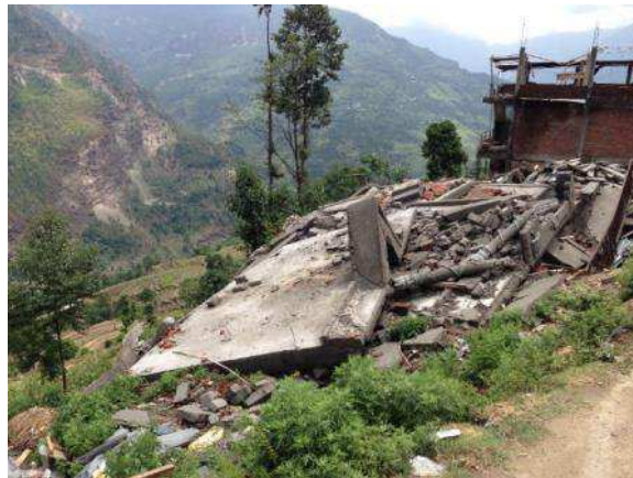
Figure 3.26. Collapsed concrete frame brick infill house in Maneshwor
