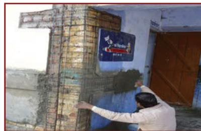
Full height wall to wall separation being rectified with WWM corner splint and additional straps.
