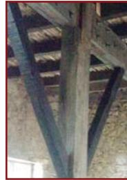
Make the end connection of bracing strong as shown in sketch below. Pre-drill pilot hole to prevent splitting of wood. Adopt same design at other end.
