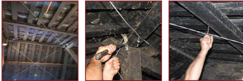
1. Install GI wire diagonal ties on underside of the roof with tie ends connected to roof timber.
