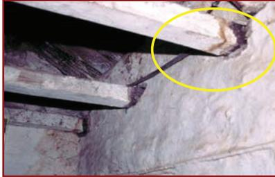
Sliding out of timber joists sitting on walls
