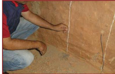
4. Using plumb-bob and cotton string mark the alignment of wires in the upper story. Continue up to attic in the same manner.
