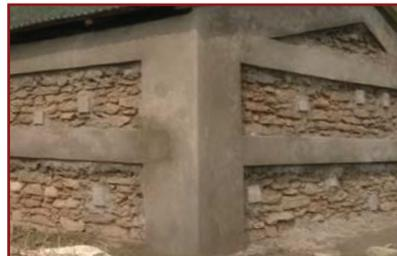
12. Cover splints with 1:3 cement - coarse sand plaster in two coats exactly as is done in the belt and cure for 15 days.
