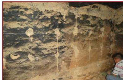
2. Divide space between belts, and also between the mid-height/sill belt and floor line in parts not wider than 400mm (16").
