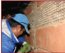
4. Use pliers and twist the free ends of cross-link 3 times keeping vertical wires between the ends.
