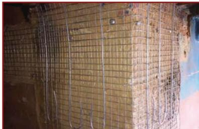
11. To ensure continuity of WWM with upper storey, at the top end under the ceiling, install 4-4mm wires on each leg with 600mm overlap plus 150mm long hook, and extend up to storey above
