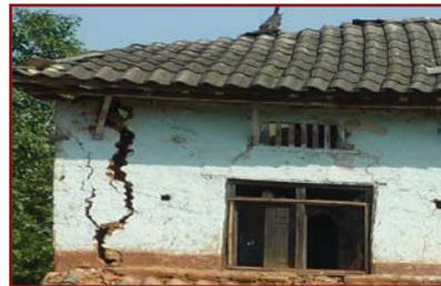
Vertical cracks developed at corners because of poor wall to wall connection.
