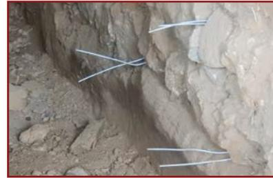
2. Insert cross-links in holes. **Be careful of cross-links protruding out and protect eyes from injury.**
