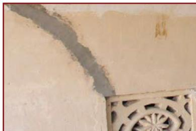
3. If structure has cement mortar and/or cement plaster then seal crack with 1:3 cement mortar after wetting the crack surface and cure it for minimum 7 days.
