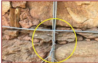
3. Each horizontal wire is anchored to all vertical wires it crosses using 1mm GI binding wire. Keep the wire as level as possible.
