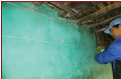
**3. With top edge of belt marked, next mark the bottom line of the belt** on all four walls to get the desired width 300mm of the belt
