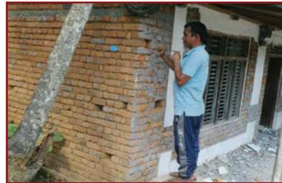
2. Install shear connectors a day before the splint installation. Continue to cure until splint is plastered. Exercise care not to exert too much force on shear connector while splint installation.
