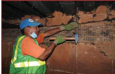
3. Mark the exact location of the vertical wires on the underside of ceiling. Drill hole through the floor.
