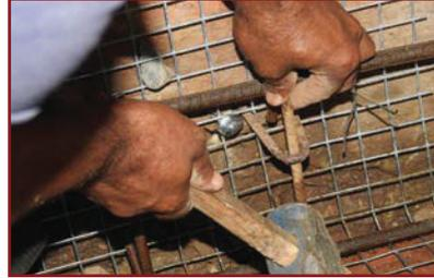
8. Anchor the cage to the wall with 6mm U shaped anchors 150mm long hammered in to the masonry joints to hold down the reinforcement tightly.
