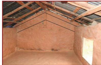
13. Mark Gable belt 150mm (6") below the top edge of the gable wall. while ensuring the proper connection with attic wall Eave belt.
