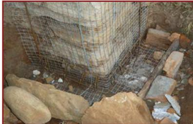
9. Install form work not exceeding 150mm in width from the steel cage to prevent wastage of concrete.
