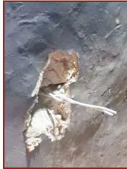
6. Make sure open ends of cross-links protrude out from the wall on both faces.
