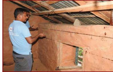
11. Measure the width of the Eave belt from top line of the belt and mark bottom line of the belt with the help of the tube level.
