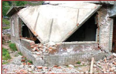
Consisting of wide crack with a portion of the slab bent resulting in bending and exposing of reinforcing bars.
