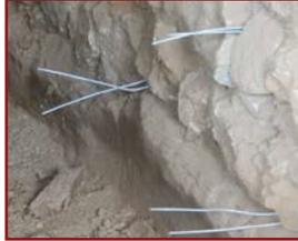
1. Install cross links at the junction of vertical and horizontal wires starting from 75mm above the floor
