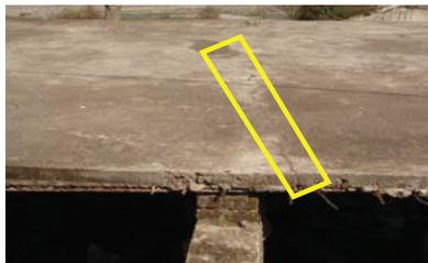
Grade1/Grade 2 Crack in RC roof/floor
