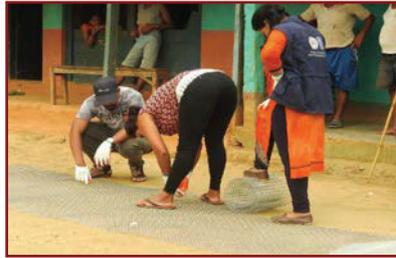
1. Cut WWM of required width and 400mm longer than the required length, while ensuring minimum waste.
