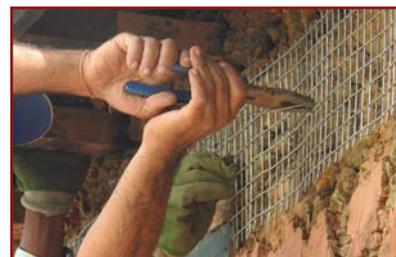
6. Pull out the cross-link ends in such a way that they catch at least two wires of WWM and twist them three times max to tightly anchor the mesh.
