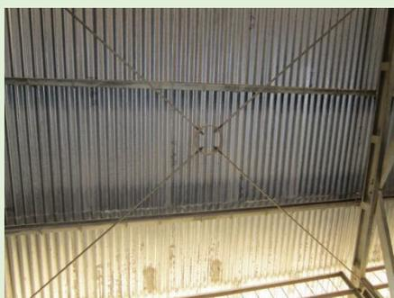
Steel bracing to roof
