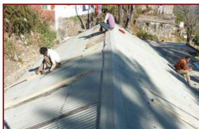
Nails being replaced by 'J' hooks to anchor tin sheets to purlins.
