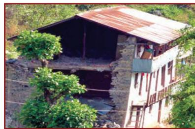
Roof and intermediate floors need to be jacked up, front and rear walls to be dismantled in step like manner, the end wall to be rebuilt all the way to roof such that it is well connected to side walls, and anchored to timber floor and roof
