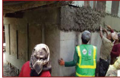
16. While still wet, apply neat cement slurry followed by first coat of cement: coarse sand (1:3) plaster of 12mm (0.5") thickness.
