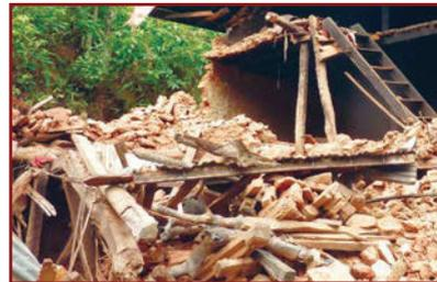
Falling debris from the upper storey or attic causing damage.
