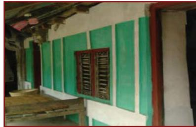
18. Finish belts and splints as desired. All vertical and horizontal wires may be covered with 2" (50mm) wide strip of cement plaster or can be left exposed.
