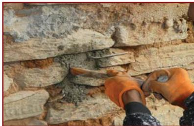
4. Next fill the entire hole to encase the rod with concrete while continuously compacting it with a rod
