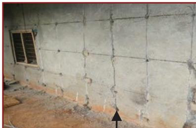
1. Take the level 75mm (3") above the finished ground floor as the datum and mark horizontal line on the out side face of the wall. It indicates the location of the bottom most wire.
