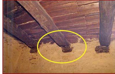
Sliding of timber joists sitting on bearing stones projecting out from walls.
