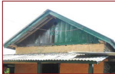
19. Alternatively replace masonry gable with GI sheet or timber on timber frame.
