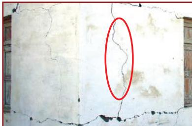
Grade 2 cracks in wall with Cement plaster.
