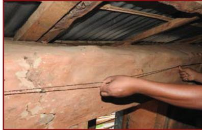
10. Mark the top line of Eave belt with string 150mm (6") below top of the wall. Follow the same on all four walls inside and out side using tube level.
