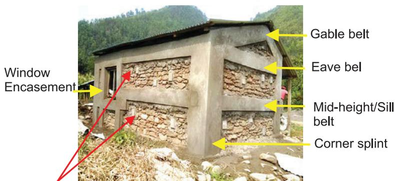
Horizontal and Vertical CR wires are to be installed in the spaces left uncovered by the belts and splints.
