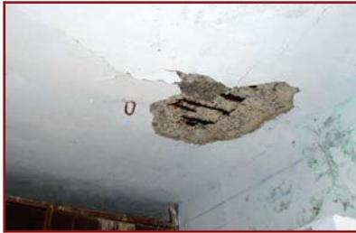
2. Dry clean the concrete surface to remove all loose materials.
