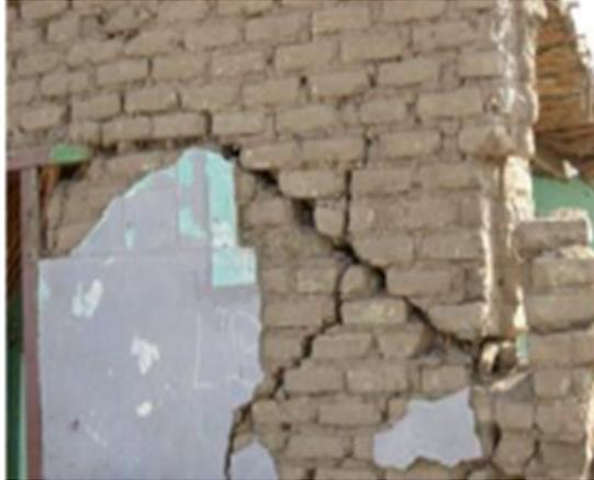
**Figure 7: In-plane damage in wall**
