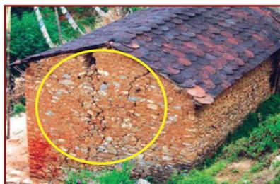
Dismantle the cracked walls further in step like manner all the way from ground level, while propping up the roof and floor. Rebuild walls to connect well with adjacent walls, floor and roof
