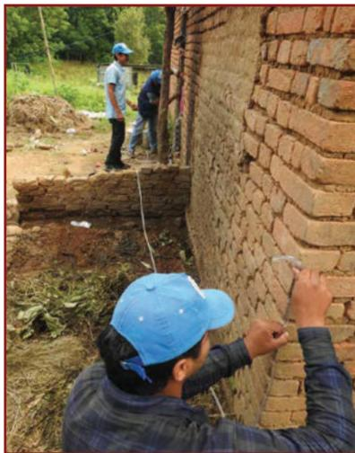
7. Using the tube level mark the top and bottom line of the belt on the outside walls, ensuring same level as on inside walls.
