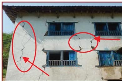
Grade 3 cracks in plastered wall
