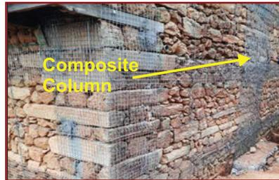
8. When belt length is greater than 5m then install Composite Column as per specifications at the mid-length of belt.
