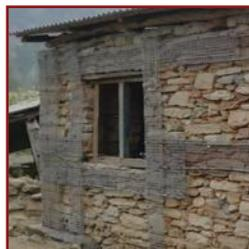
2. Install the prepared mesh in right location with right overlap with Lintel & Mid-Height Belts.
