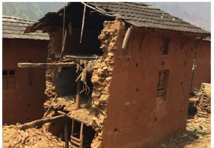
Figure 4: Collapsed gable wall
