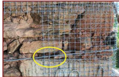
4. When a wire goes over and across the Splints it should be tied to Splint at minimum 3 points with 1mm GI binding wires.
