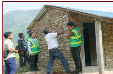
**4. With the tube level follow the same level and mark the top and bottom line of the belt on the outside faces of walls.**
