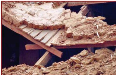
Breaking of floor joists
