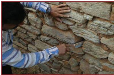
2. Make small hole approx. 100mm X100mm (4”x4”) and 250mm (10”) deep by removing stone at desired location. Clean the hole with wire brush and water.
