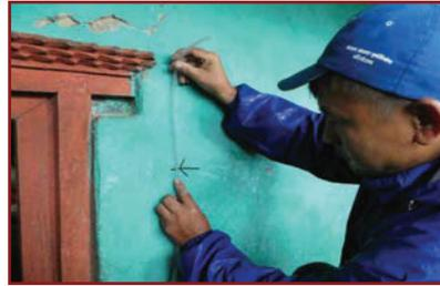
2. Simultaneously start marking the opening encasement on the sides of openings. Use plumb bob and mark vertical lines. Follow the same lines on both faces of the wall. Once lines are marked, mark the location of cross links as per the specification.
