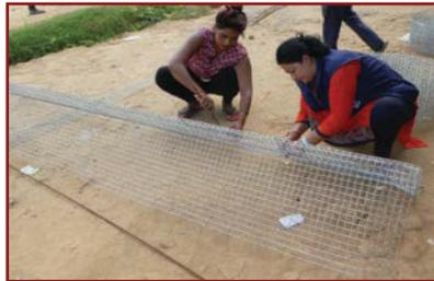
1. Make WWM straps 800mm wide for L and 400mm wide for T junction for full wall height with 450mm extra for starting below plinth level.
