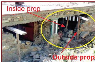
Props placed inside as well as outside the building to support the slab
