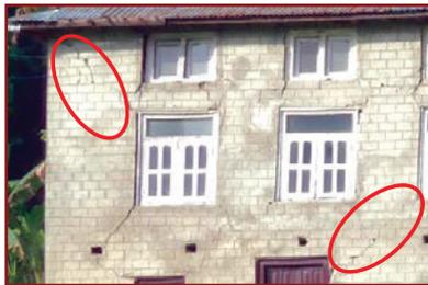
Exposed masonry wall having Grade 2 cracks
