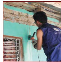
Use electric grinder or chisel and cut the plaster precisely within the area marked for the measure to prevent excessive plaster removal.
