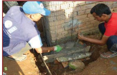
10. Pour 1:1.5:3 concrete continuously rodding to prevent cavities in concrete. Cure concrete for 15 days.
