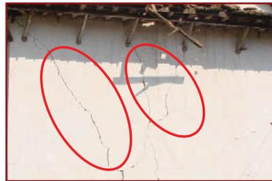
Grade 2 cracks in Cement plastered wall
