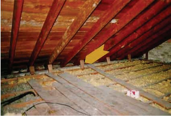
R.4.1 view inside the attic showing the rafters and the absence of collar beams and joist connections to the rafters
