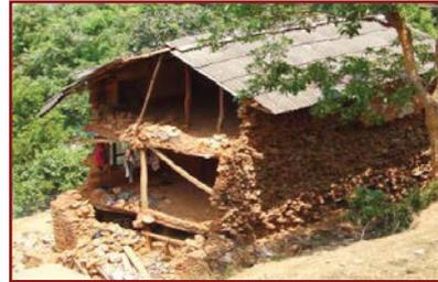
Parts of wall or full wall collapsed because of poor wall to wall connection or the walls were too long or too high
