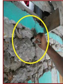
7. Insert small stones or stone chips below and above the cross links using little mud mortar for closing the hole.
