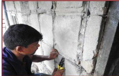
1. Install horizontal wires on both faces of walls in the portions not covered by the belts. Stretch each horizontal wire around the walls and corners.
