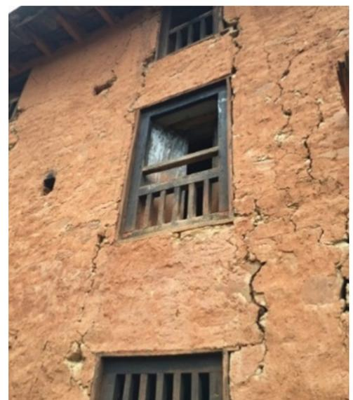
**Figure 6: Diaphragm deficiency**
