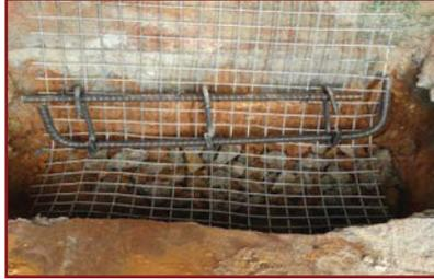
7. Place 10mm dia steel bar cage with weld mesh end projecting out 150mm at the bottom. All hooks of the cage must be bent away from the wall.
