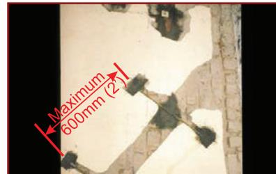
Hammer in 'C' clamp at maximum distance of 900mm in the mortar joint perpendicular to the crack
