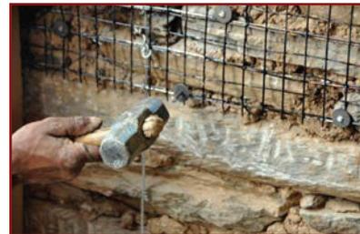
4. Hammer in 100-150mm (4"- 6") long masonry nails in mortar joints in zig-zag manner at 300mm spacing to anchor the belt securely to the wall.
