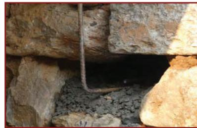
3. Fill bottom half of hole with concrete (1:1.5:3) and place ‘L’ shaped rod over it with the hook end inside the wall.
