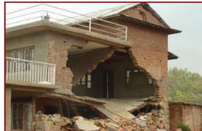
Floor collapse because of collapse of wall and poor floor to wall bonding.
