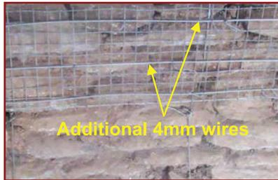
7. Install 4mm wires having 150mm (6") long hook at their ends using 1mm GI binding wires on the WWM belt as required per specifications
