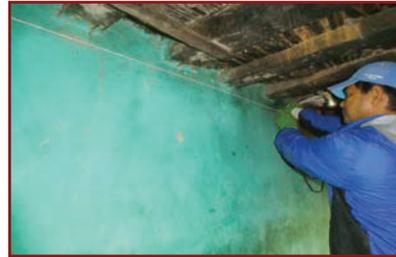
**2. Consider this level as the datum.** Use the tube level to get the correct level and **mark the top line** of the belt on all four walls with cotton string. The belt alignment can be above or below this datum depending upon the obstructions like beam, window etc.
