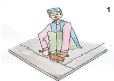
1. Clean the crack with wire brush.
