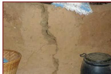
4. If the structure has mud mortar or mud plaster then seal the crack with mud
