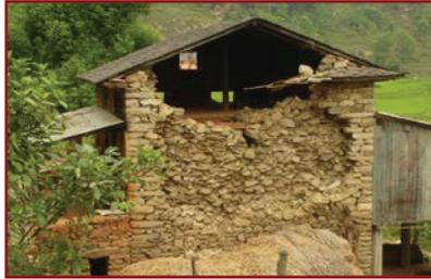
Separation of a face followed by delamination of part of a stone wall
