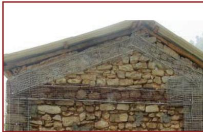
18. Install gable belt with its top edge approximately 100-150 mm below the top edge of gable wall.
