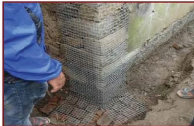
3. Rake all the mortar joints and Install WWM splint starting from 450 mm below plinth level and continue through to the top of the wall at roof level.
