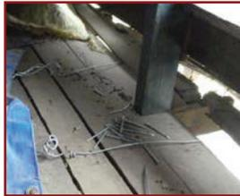
7. Pull up wires along both the faces of wall and over the wall plate or portion of the timber floor of the hybrid structure (in which the upper storey is made of tin and timber, and is placed on top of the masonry structure), and anchor it to the wall plate with heavy nails.
