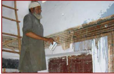
15. Splash the exposed wall surface with water to remove all the dust as also to make it moist.
