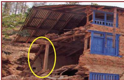
1. Prop up damaged floor, and clear all the debris on it, if any.
