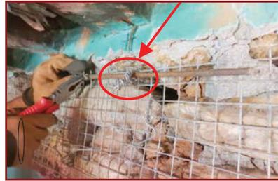
2. Anchor the cross-link with a 10mm diameter 300mm long bar installed against the outer face of the wall.
