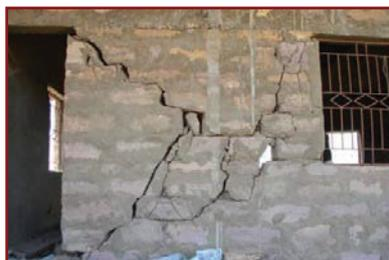
Grade 3 cracks between opening
