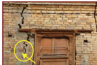
Grade 3 cracks in un-plastered wall
