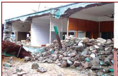
Undamaged RC slab on severely damaged wall
