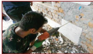
1. Remove plaster to locate joint in masonry. Make around 15 mm holes in joints with help of a short pointed end 'L' shaped 12mm steel rod through the wall at all locations for cross links.
