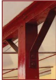
Make the end connections of bracing strong as shown in sketch below. Pre-drill pilot hole to prevent splitting of wood.
