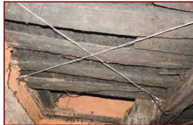
4. Install in-plane diagonal tie in 'X' configuration made of 4-2mm GI wires in each tie pulling wires tightly .
