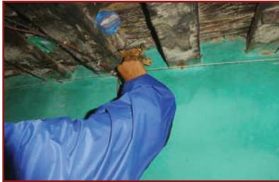
**1. Mark the top line of Lintel belt** just under the floor joists on an inside wall, while ensuring that it clears the bottom of most of the floor joists. Disregard the bottom of the beam that supports the floor joists which is significantly lower.
