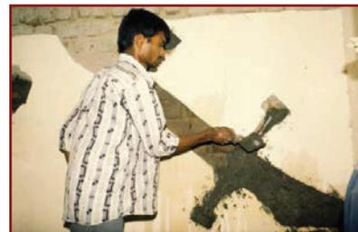
Plaster over the clamp and crack with two 12mm coats of 1:3 cement plaster.
