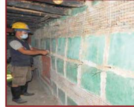
3. Stretch wires vertically and anchor on both wall faces at same time to each cross-link in row.
