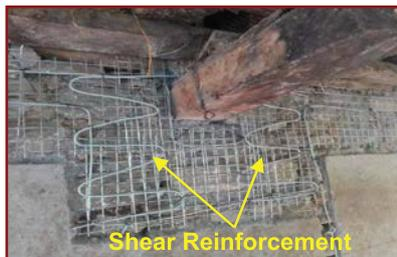
10. Shear Reinforcement installed at a change in alignment of Eave belt.
