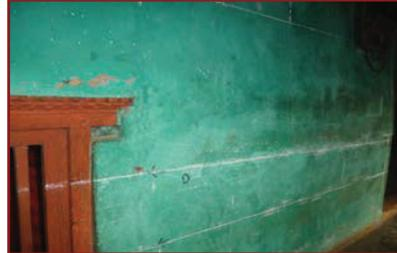
6. Mark the top and bottom line for this belt measuring from the top edge of the Lintel belt. Do not measure from any other point. Use tube level to ensure the right level of the belt along its full alignment.
