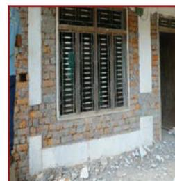
Rake all the mortar joints to the depth of 12mm (1/2") by hand using chisel. Clean the surface with wire brush and water.
