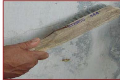
2. Clean crack with wire brush to remove all loose materials including dust.
