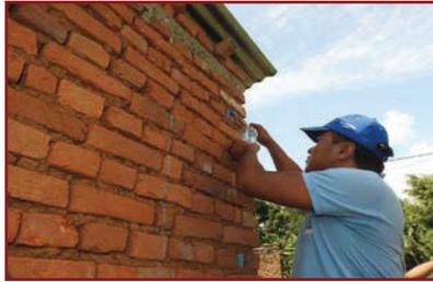
1. Start marking the vertical splints at 'L' and 'T' wall to wall junctions. This is installed only on outer face of walls. Use plumb bob for marking vertical lines. Once lines are marked, mark the location of shear anchors as per the specification.
