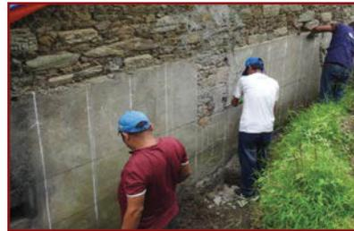
1. Vertical wires are to be marked in the space between a splint and an opening encasement or next splint. Start with the ground story. Moving from one end of wall mark the first and last lines on a wall 100mm (4") from the splints or opening encasement. Measure the gap between these lines and divide it in vertical spaces no wider than 400mm to mark the wire locations. Use string and plumb-bob for marking.
