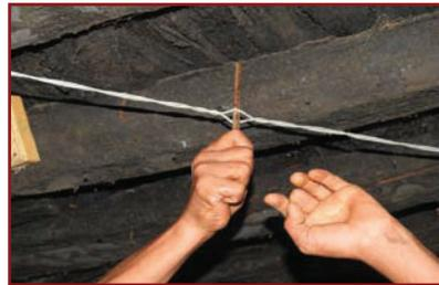
6. Pre-tension each Tie by pulling at the time of installation followed by twisting. Excessive twisting can break the wires.
