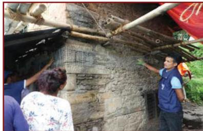
3. Install the prepared WWM on the raked and clean wall surface where the cross links are pushed in and anchor it with nails first.
