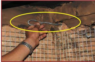
1. Install special cross-link made of 2-2mm wires folded at mid-length to make a loop at one end in four corners of each room through masonry walls .
