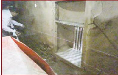
5. Mark Sill belt under the window if sill is 600mm (2') or higher. Otherwise at approximately 900mm (3') from the bottom of Lintel Belt or close to mid height mark the belt. If window is close to the floor, discontinue the belt or continue a smaller width belt under the window.
