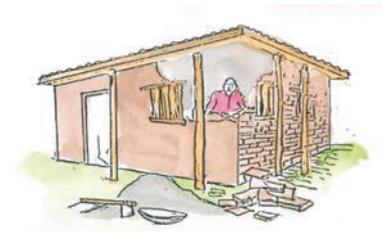
**Systematically propping up slab, removing portions of damaged walls, and rebuilding them portion by portion one can save the RC roof. Advise from an engineer is recommended.**
