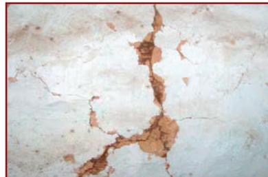
Grade 2 cracks in wall with mud plaster
