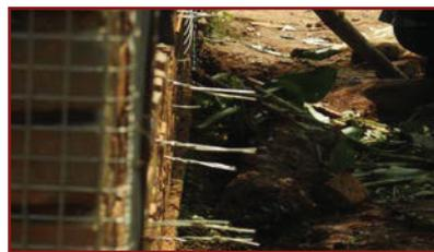
3. The holes shall be just large enough for inserting the cross links through full thickness of the wall.
