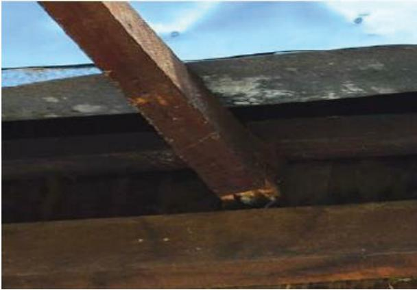
R.3.1 Purlin detached from rafter due to inadequate nailing
