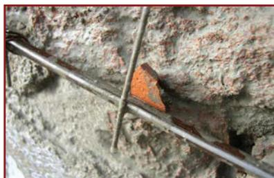
5. Provide 15mm (0.5") thick spacers of any suitable material between the wall surface and the mesh to ensure full encasement in plaster.
