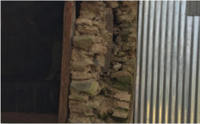
Figure 1: Cross section of a damaged SMM house showing the dual layer of stones
