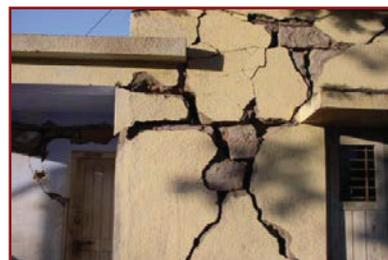
Grade 3 cracks in masonry
