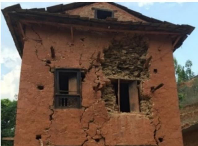
Figure 3: Short wall out-of-plane damage in SMM building
