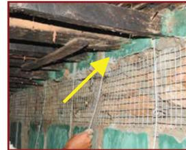
6. Continue vertical wire through a hole in the floor to go over the eave level wall keeping it taut all the time.
