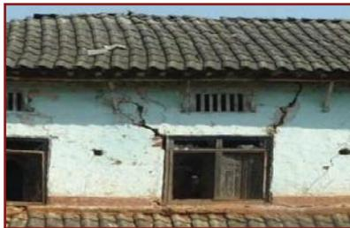
Large diagonal cracks developed at the door and window because of the absence of a band at lintel level.
