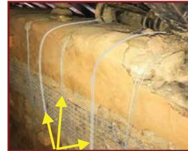
8. Pull wires from inside and out side faces over top of attic wall and anchor to cross-link on the opposite face below the belt.
