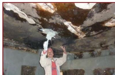
Spalled concrete removed, rusted bars cleaned and coated with anti-rust chemical, bonding agent applied and finished with micro-concrete.
