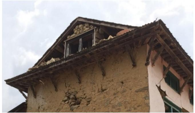
Figure 2: Damaged gable wall in an SMM house
