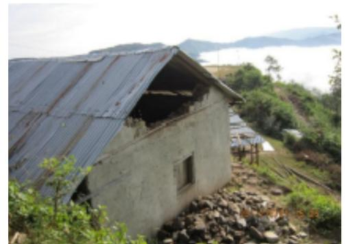
**Figure 5: Attic wall out-of-plane damage**
