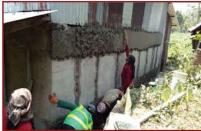
17. After 1 to 2 hours, apply second coat of plaster with same mix and with enough thickness to provide 20mm cover over the GI wires.
