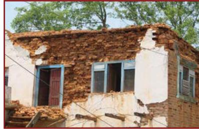
Delamination of a thick brick wall
