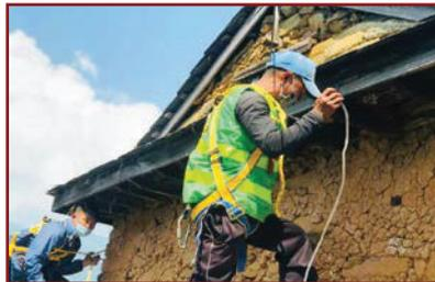
12. Finish marking attic wall Eave belt on out side wall also using tube level ensuring the same alignment.
