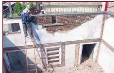
Damaged brick masonry wall being rebuilt to reinstall RC slab on it.
