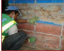
2. Starting from each bottom most cross-link attach 1-4mm GI wire on both faces of the wall.
