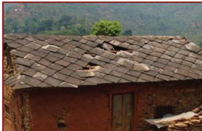
Roof damage because of degraded timber and dislodged slate.
