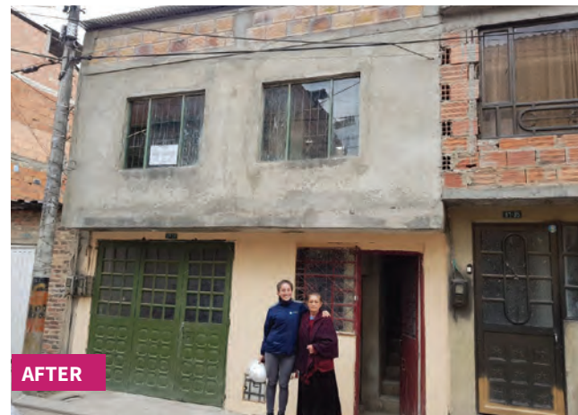
Added ring beam, confining elements, plaster and mesh plaster, upgraded roof, and improved sanitation
