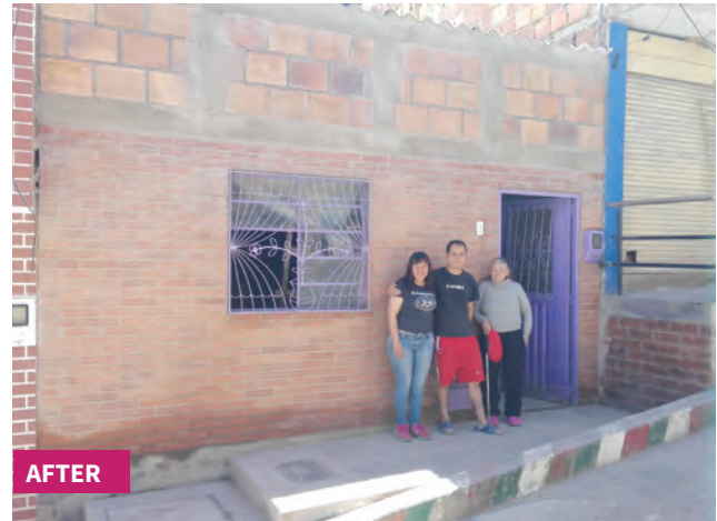
Added ring beam, confining elements, and plaster, and improved roof and sanitation
