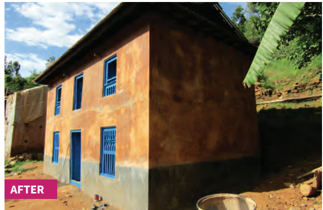
New ring beam, through ties, strongbacks, slab strips, plaster, stone gable infill replaced with lightweight timber panels, and improved roof 12
