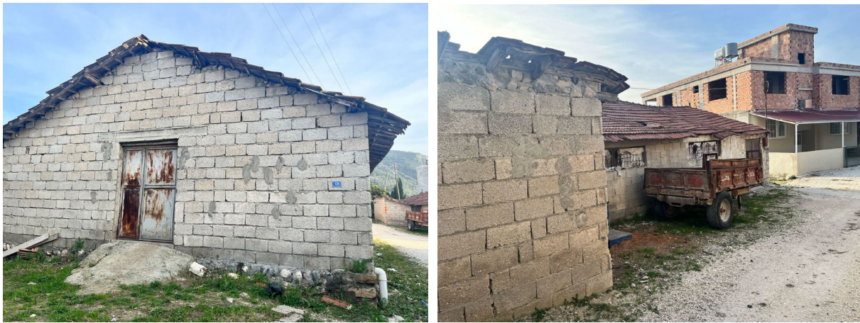
FIGURE 15 Unreinforced block masonry buildings in Balıklıdere village, Hatay
