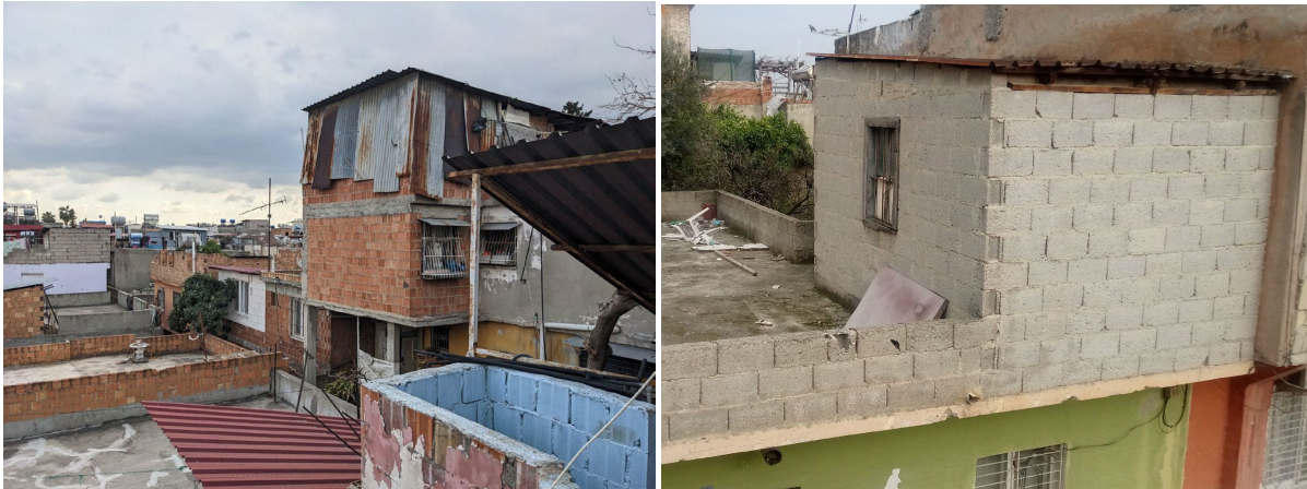
FIGURE 13 Unreinforced masonry in urban areas (Adana)
