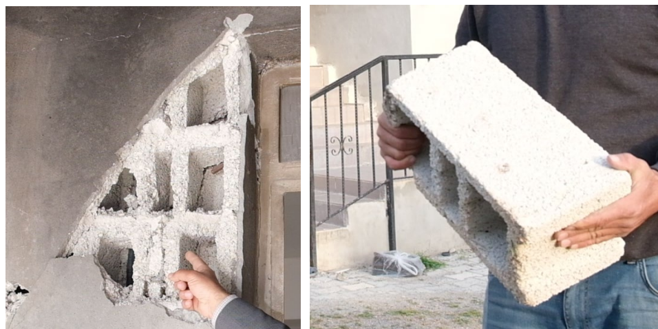
FIGURE 18 Pumice concrete blocks used as structural material in unreinforced masonry buildings and as non structural material in the infilled walls of RC Frames.
