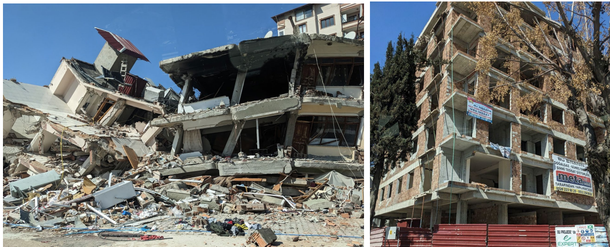
FIGURE 11 RC shear walls and beam-column frames in urban areas in Antakya, Hatay
