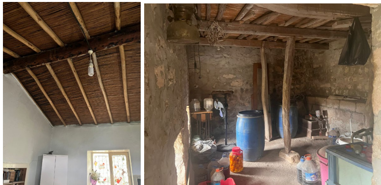
FIGURE 17 Roof and floors of an unreinforced stone masonry house in Vakıflı Village, Hatay. Pictures of a one-story house. The figure on the left shows the roof at the first floor and the figure on the right shows the basement.
