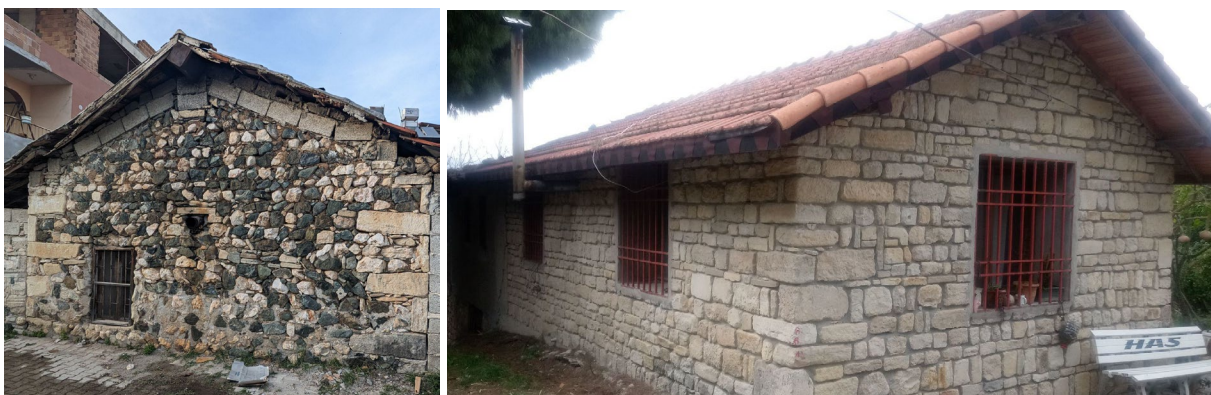
FIGURE 16 Unreinforced stone masonry buildings in Balıklıdere and Vakıflı villages, Hatay
