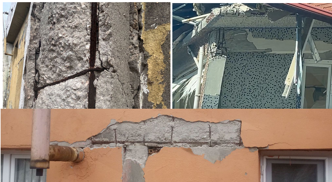
FIGURE 21 Poor concrete quality and reinforcement detailing
