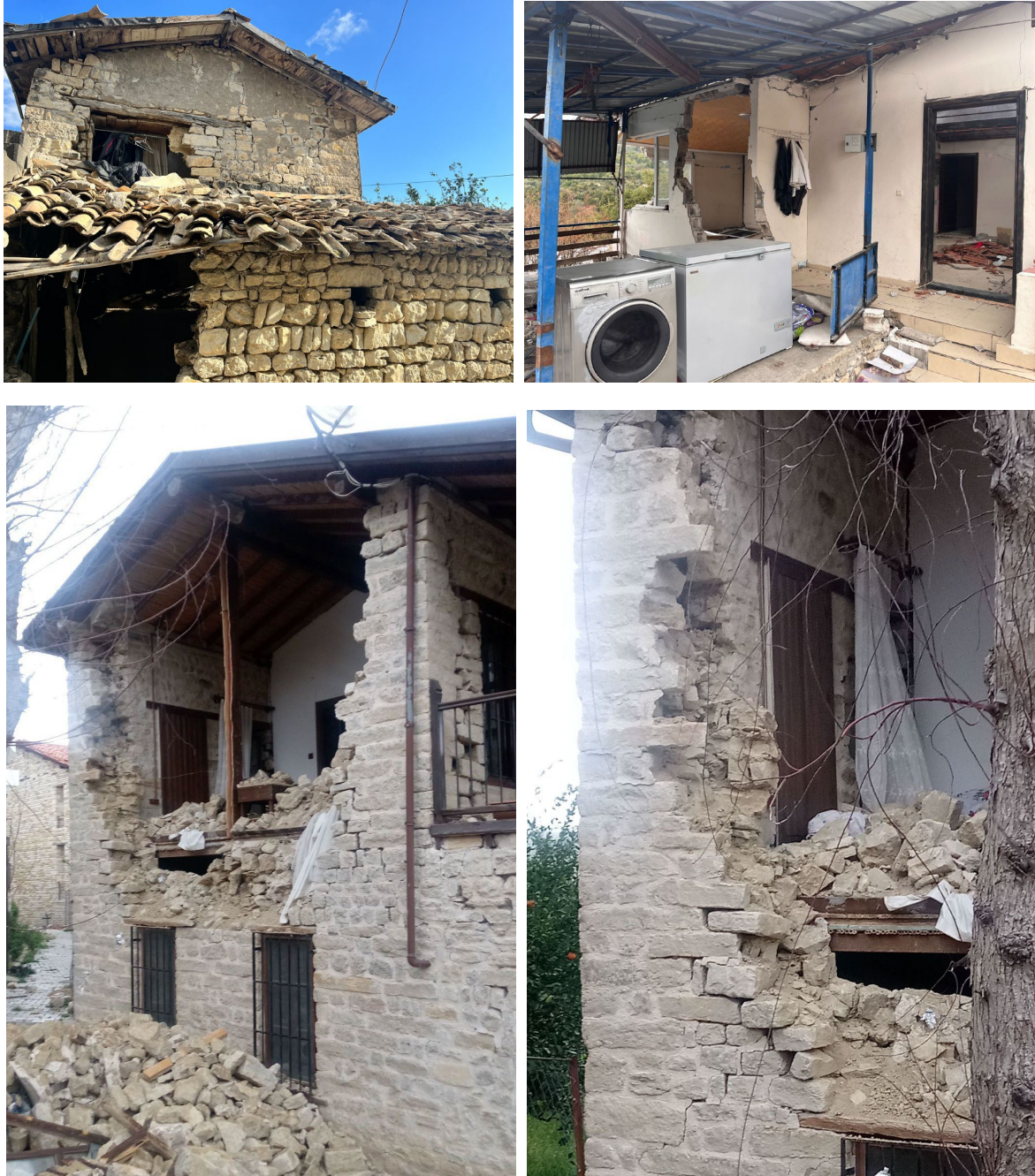
FIGURE 25 Damage assessment of unreinforced masonry buildings
