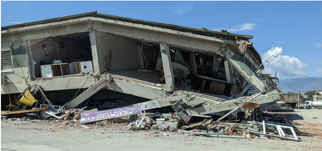
FIGURE 23 Damage assessment of non-ductile RC Frames with or without infill walls.
