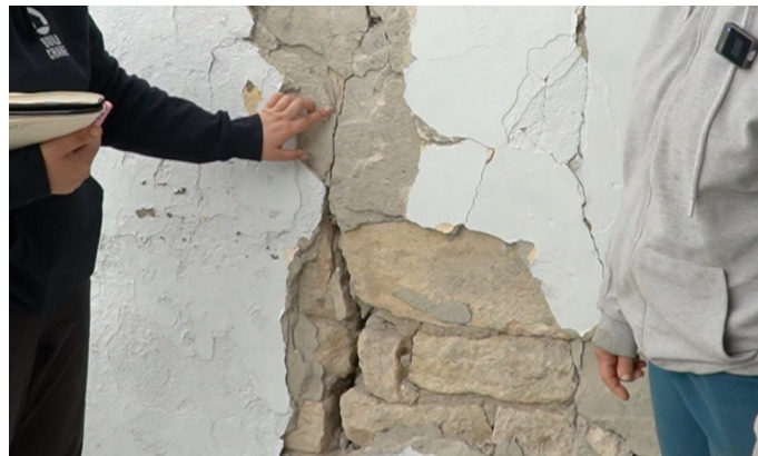
FIGURE 20 Stone masonry found in rural areas
